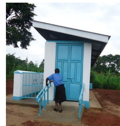
Toilet block with a specific toilet with handrails and level path. Credit: Plan International
